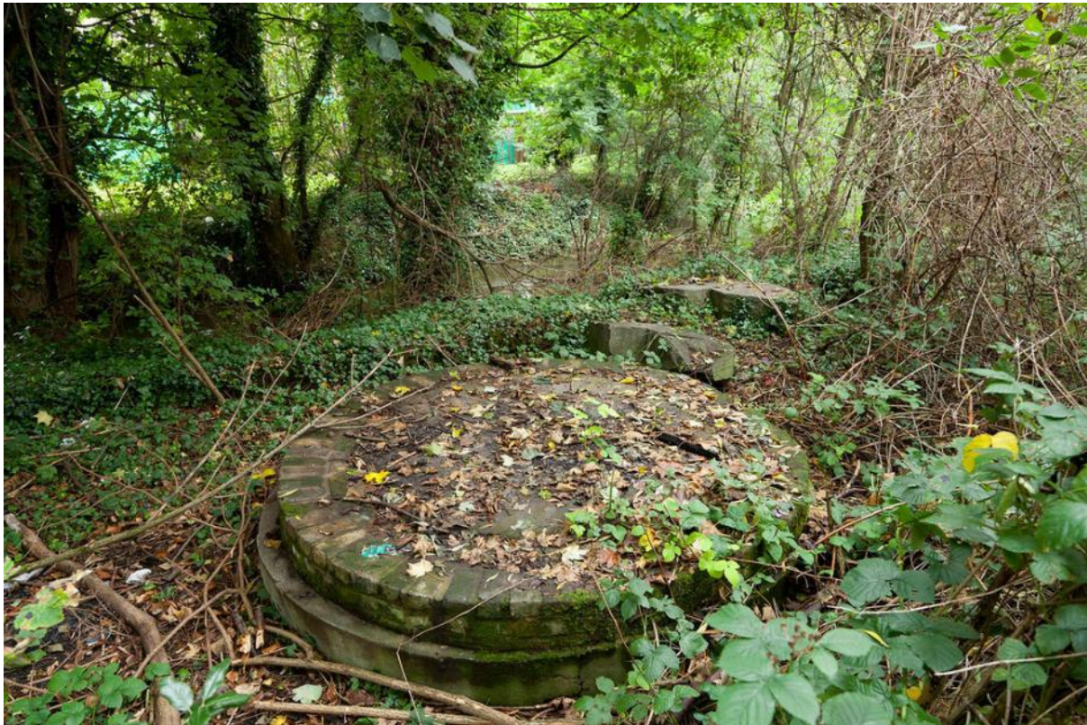
The current condition of the brick base for the base runner stone
