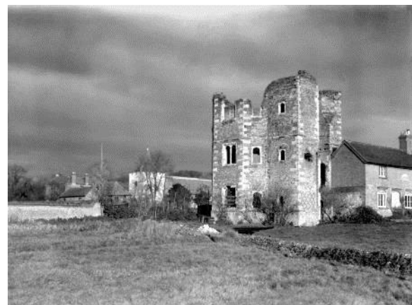
View of Otford Palace, taken in 1934 showing the ivy removed and the buildings adjoining the Tower having gained a second brick storey (Otford.info)
