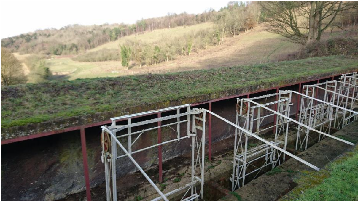
Target raising mechanisms at the southern end of the range (looking northwards up the range)
