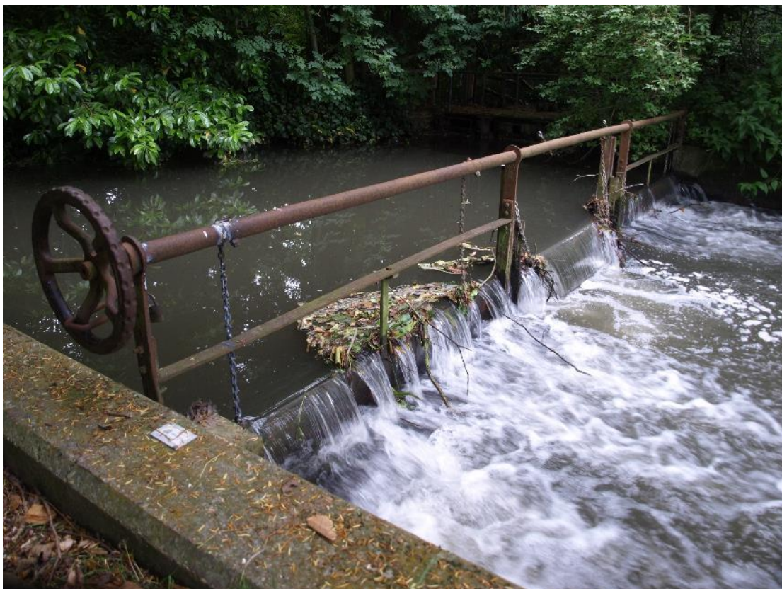
Weir structure on the River Darent near Shoreham
